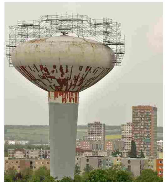
Figure 5.14 Scaffolding conforming to unique form
