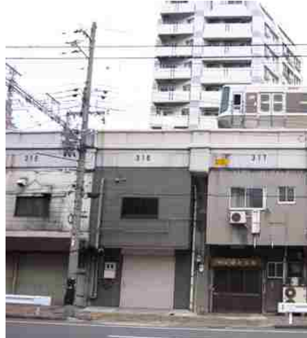
(b) (infra)structural gaps
